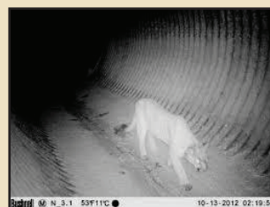
Although studies show pumas prefer more open box culverts, if an underpass connects appropriate habitat in the cat's normal travel pattern, has fencing or other geographic features to funnel them within their territory, they will use a pipe culvert also.
