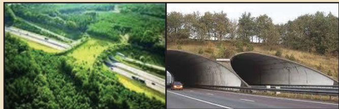
Example of a wildlife crossing overpass in Europe and Canada. Notice how you have appropriate habitat on either side of the crossing. Suitable habitat for species should occur on both sides of the crossing structure (Ruediger 2001; Barnum 2003; Cain et al. 2003; Ng et al. 2004). This applies to both local and landscape scales. On a local scale, vegetative cover should be present near entrances to give animals security, and reduce negative effects of lighting and noise (Clevenger et al. 2001; McDonald & St Clair 2004). Suitable habitat must be present throughout the linkage for animals to use a crossing structure.
